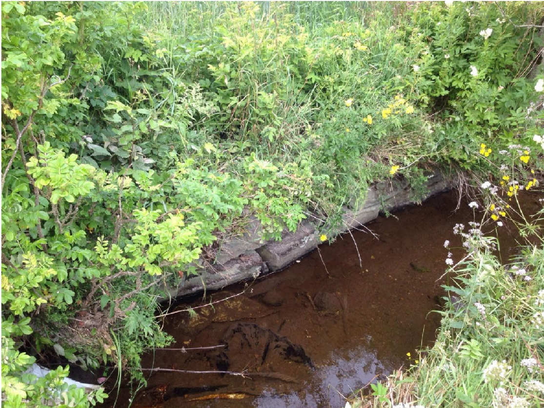
B 1- 100: Liten mur (sikringstiltak) (Placemark 16 RMo)
