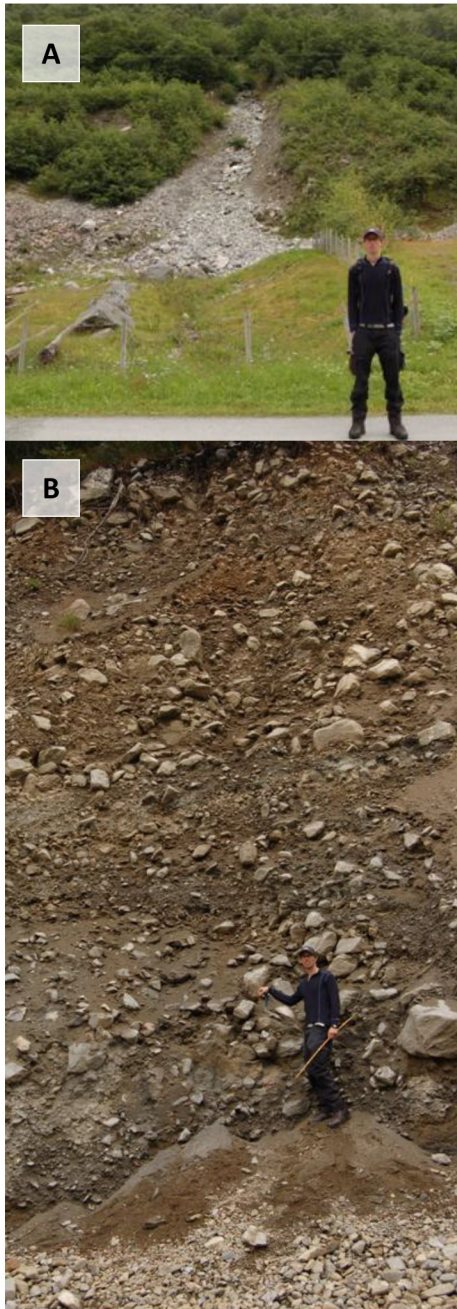
Figure 7-4: A) The lower part of Kyrkjegrova where deposits have been removed to lead new slides away from the settlement. B) Massive deposits from recurring events of debris flows, rock falls and snow avalanches 350 m north of the outermost settlement (Photos: M. Lund).
