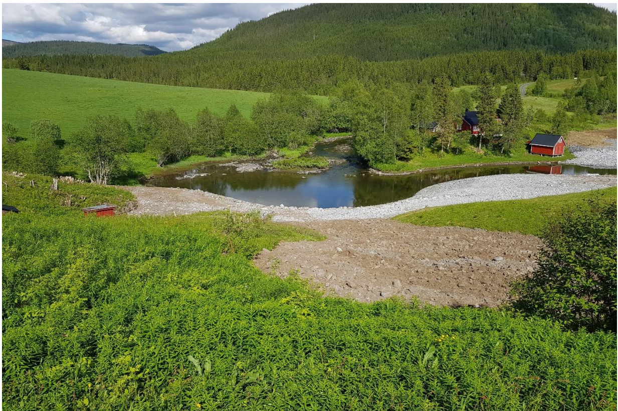
Figur: Ferdigstilt motfylling.
