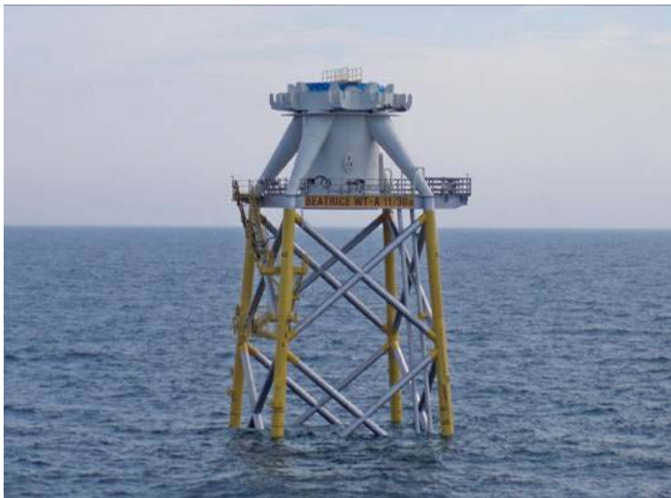
Bilde: OWEC Jacket Quattropod offshore vindturbinfundament, Beatrice
