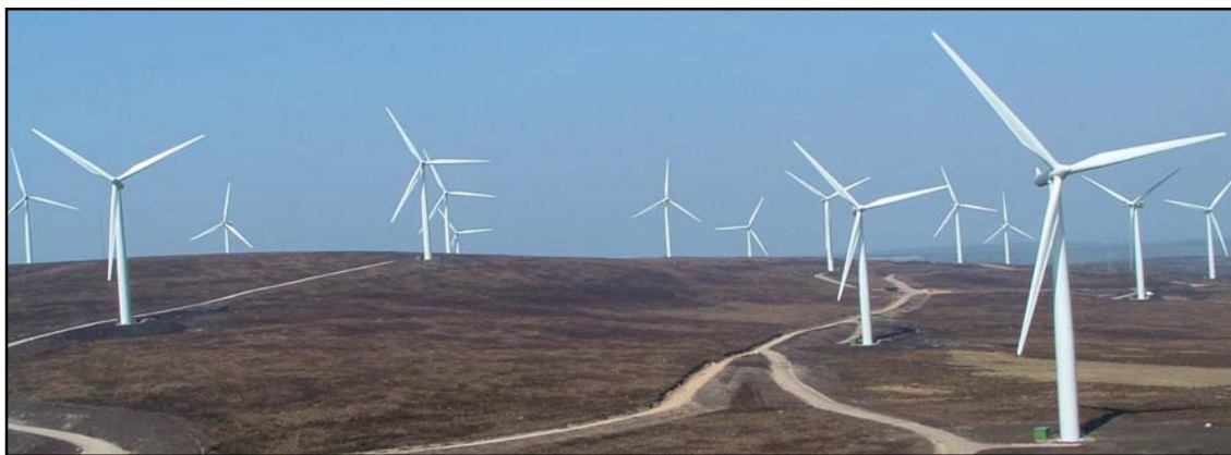
Roths wind farm, UK
