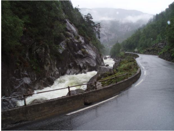
Figur 4-28: Dalelva oppstrøms Juv bru Q=9,0 \text{ m}^3/\text{s} (12.7.06)
