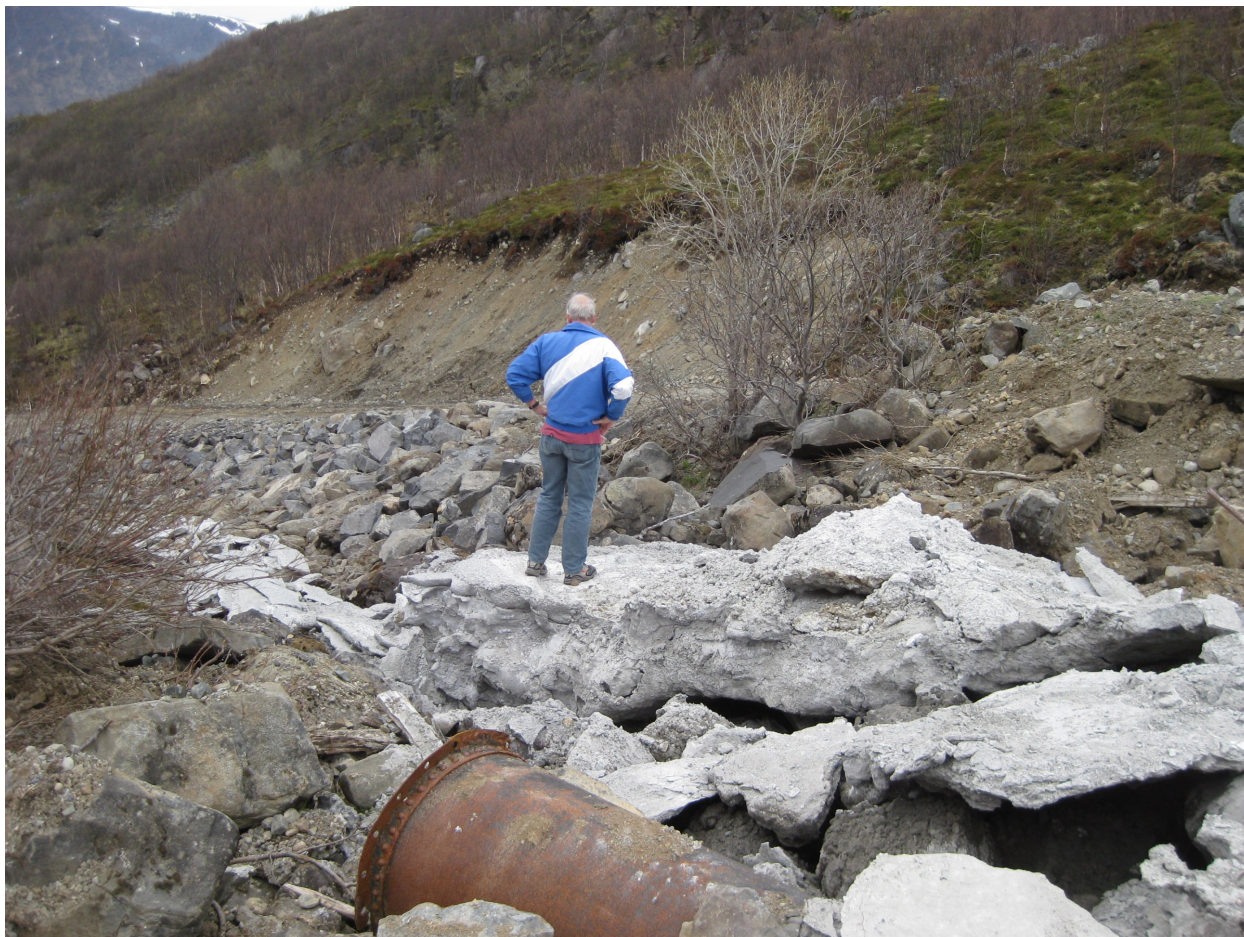
Figur 3 Betong dumpet i elveleiet
