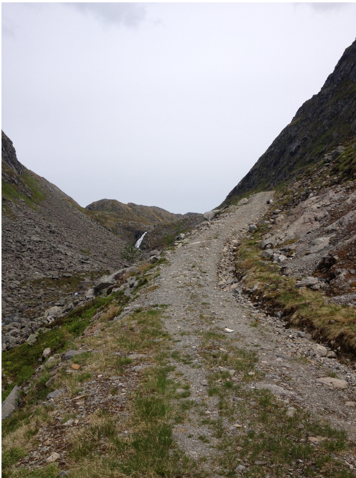
Figur 9: Sidebratt parti like ovenfor elvekryssing.
