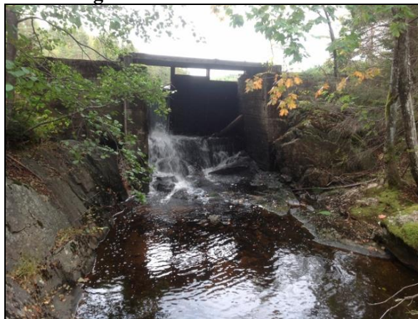
Vestre Engevannet dam
