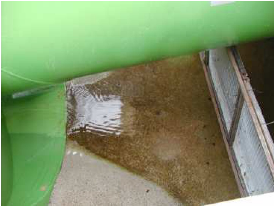
Figure 6. Intake with fish screens
