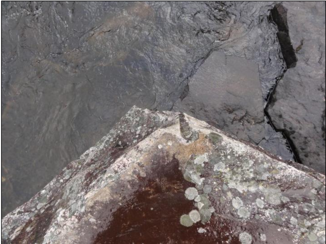
Figure 1.5. Evidence of bedrock blasting
