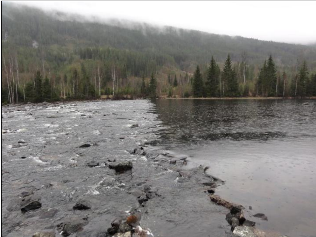
Figure 1.4. Large boulder weir structure
