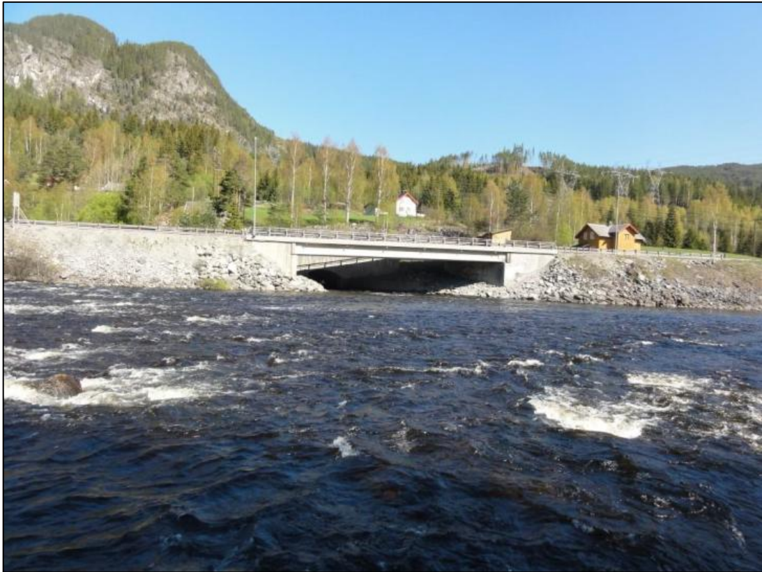
Figure 1.2. Upstream Hemsil distributary channel
