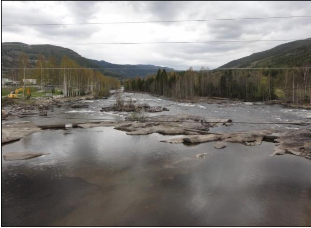
Figure 4.5. Concrete weir structures
