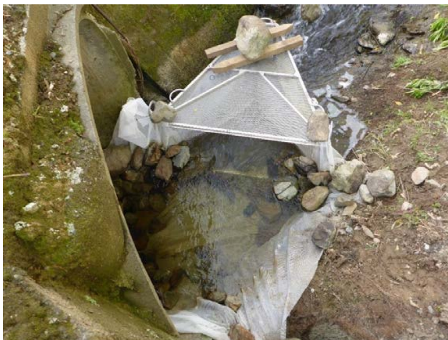
Figure 7-4: Whitebait trap installed at the culvert inlet in Kara Stream.
