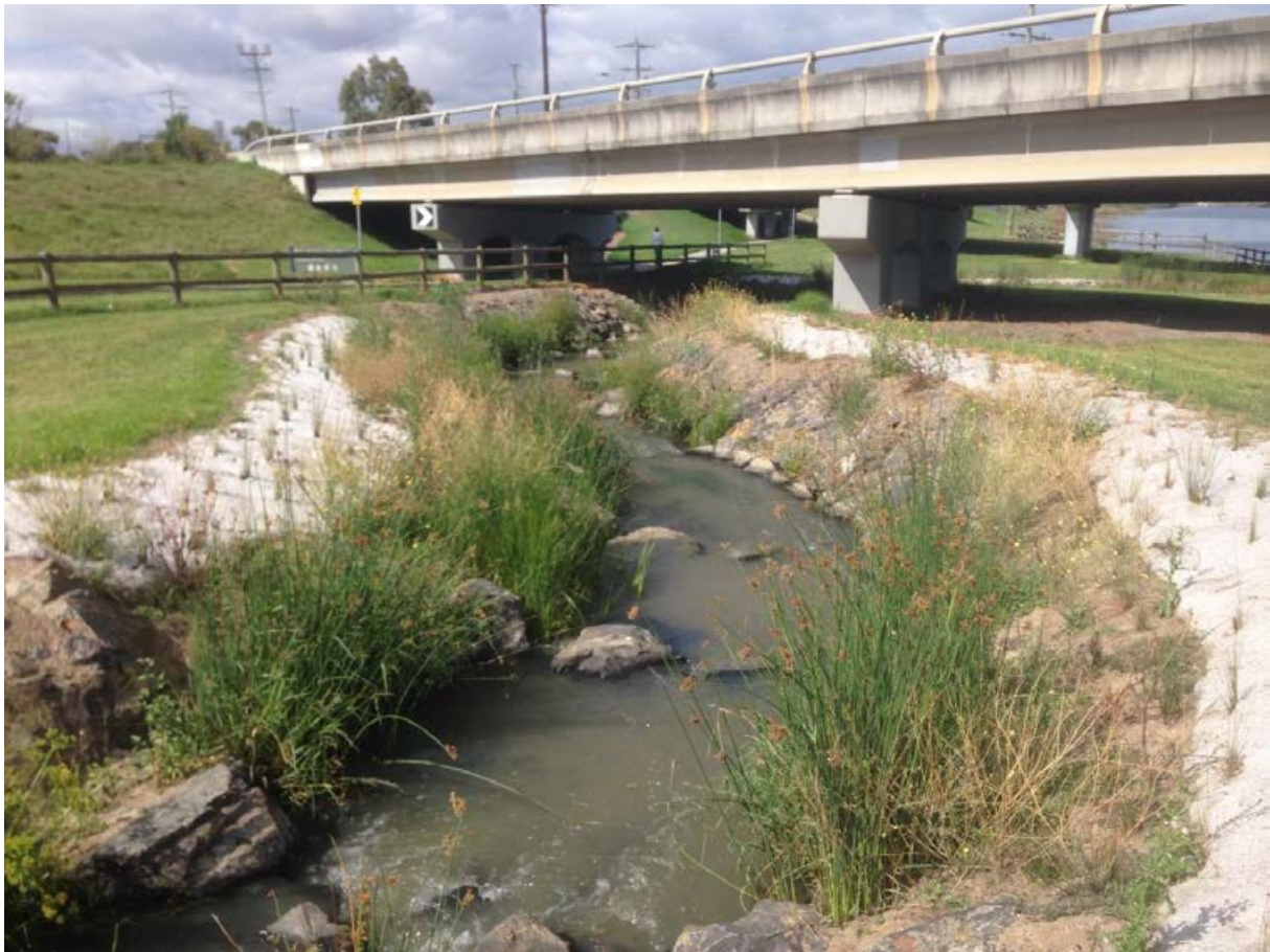
Figure 5-1: Example of a low gradient nature-like rock ramp fishway on the Patterson River near Melbourne, Australia. Photo: Paul Franklin.
