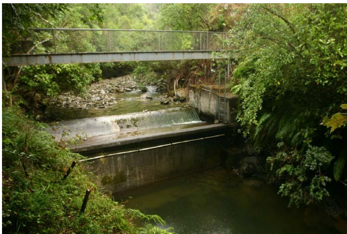
Figure E-7: An intake weir that blocks fish migrations on the Te Arai River near Gisborne. Credit: Jamie Foxley.
