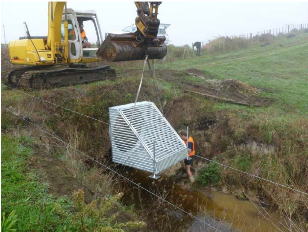
Figure 6-8: One-way gate structure prior to installation showing screen that can be lifted for inspection and clearing of debris. Credit: Adam Daniel.
