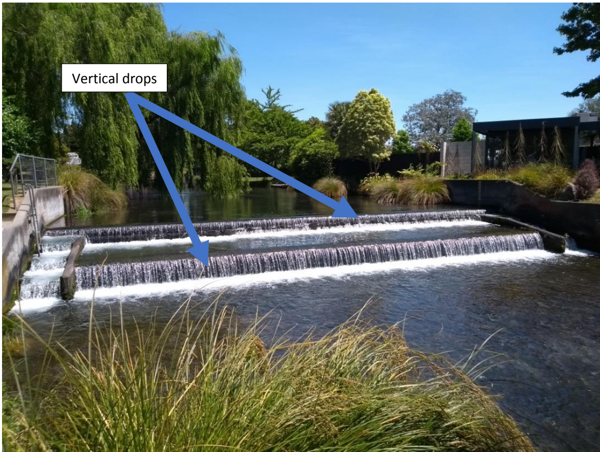
Figure E-13: Example of a weir in central Christchurch. Fish passage will be impeded by the fall height of the steps in the weir and the salmonid fish passes. Credit: Megan Brown.
