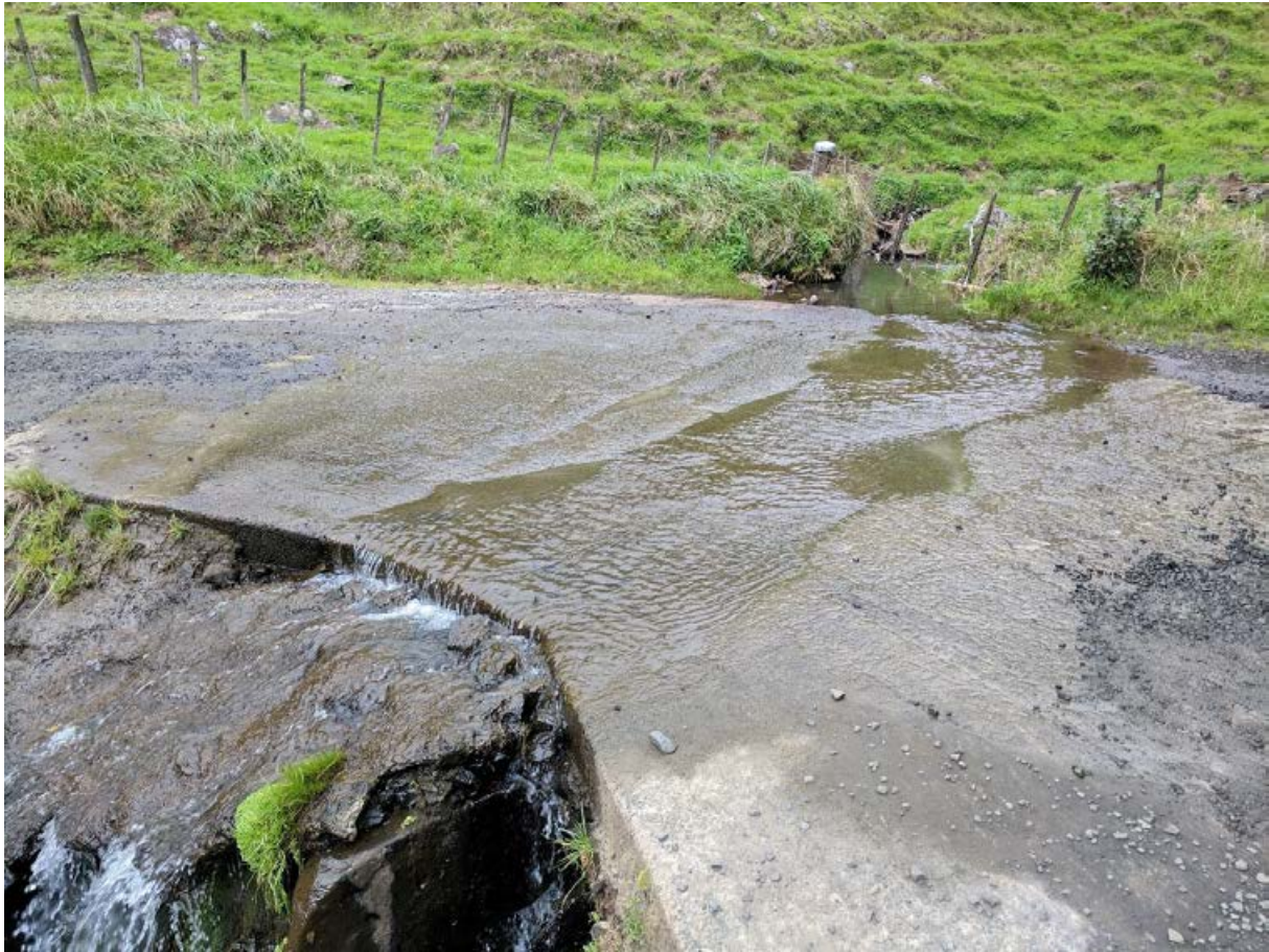
Figure E-6: Example of shallow water that can act as a barrier to movement for fish. Credit: Eleanor Gee.
