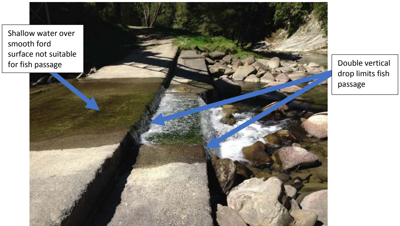
Figure E-20: Example of a ford from the Te Arai River. The fall height at the two steps on the downstream side of the ford makes a complete barrier to swimming fish species. Passage for climbing fish will be impeded by the sharp corners on the steps and shallow water across the ford, but some may access upstream habitats by taking advantage of the wetted margins to climb. Credit: Paul Franklin.
