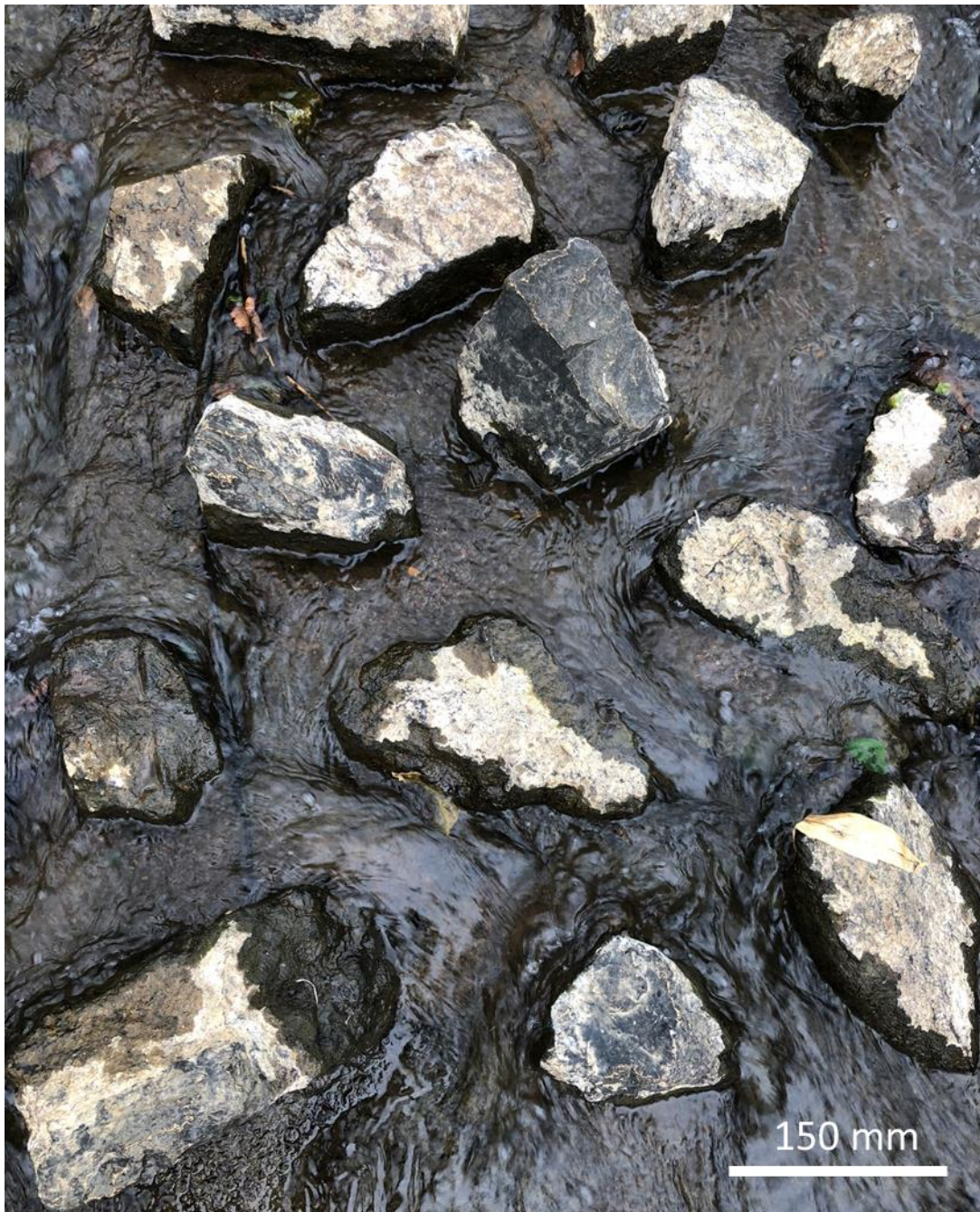
Figure 4-12: An example of rock size and spacing suitable for increasing roughness on a weir.
