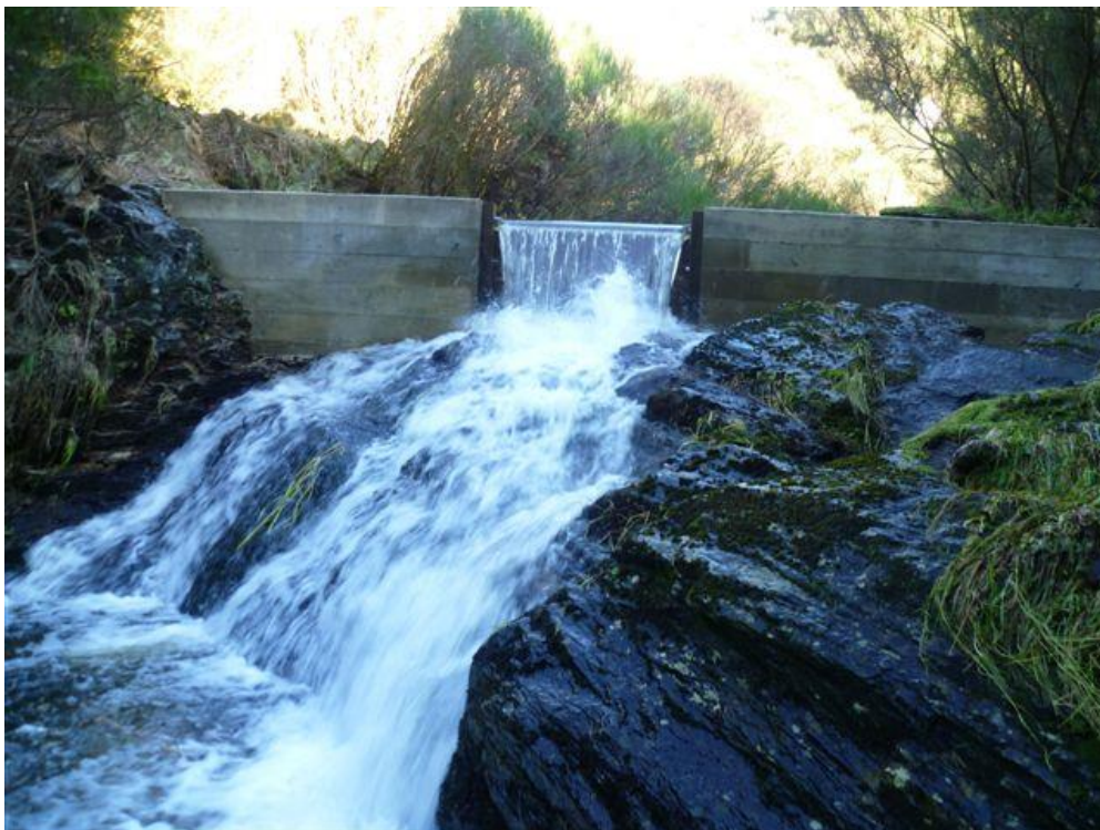
Figure 6-2: Akatore Creek barrier in Otago . A built barrier has been installed onto a natural waterfall to protect Taieri flathead galaxias, after brown trout gained access upstream when conditions changed. Credit: Sjaan Bowie (DOC).
