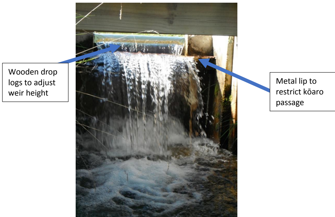
Figure 6-5: Built barrier installed in an unnamed spring of the Fraser River. The objective of this built barrier was to prevent trout and kōaro accessing a key lowland longjaw galaxias and bignose galaxias stronghold in the MacKenzie Basin, Canterbury. Key features of the barrier were the height to prevent trout access, the metal lip to prevent kōaro passage, and the wooden drop logs to allow for flushing of flows and maintenance of flows and habitat upstream. Credit: Sjaan Bowie (DOC).
