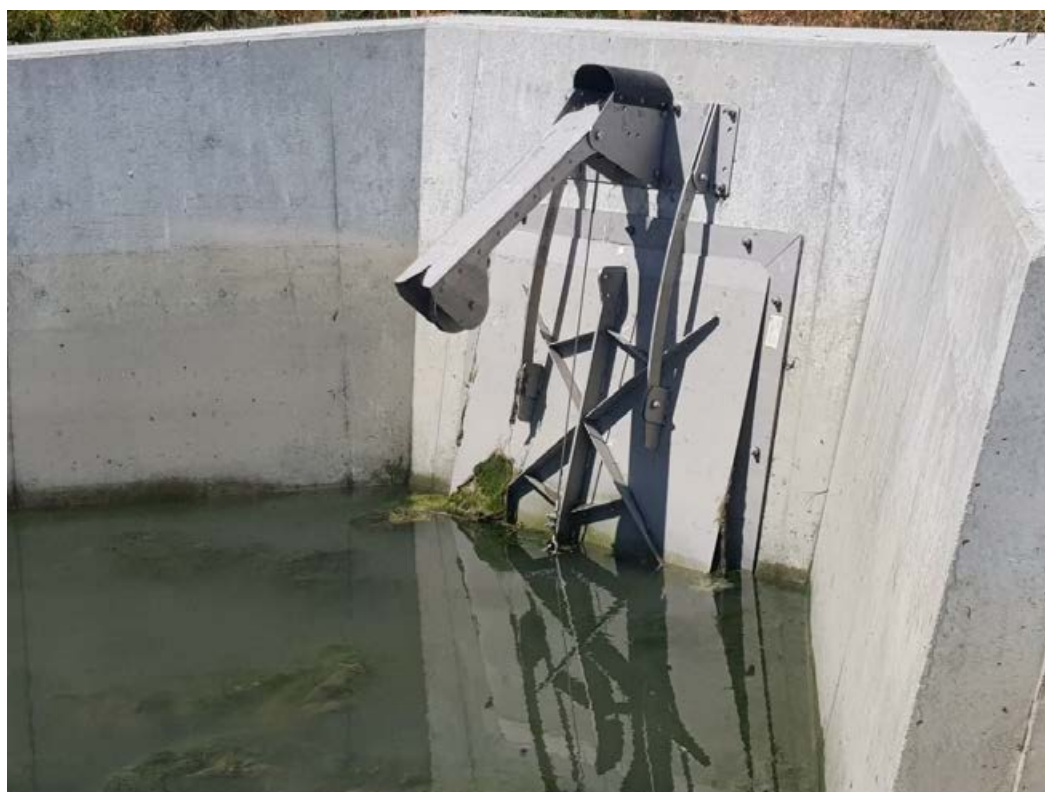
Figure 4-19: Example of a self-regulating tide gate installed in Canterbury. The counter weight system holds the tide gate open for longer on the incoming tide. The system can be calibrated to manage the magnitude and duration of the opening to best coincide with critical migration periods, e.g. the incoming tide for whitebait and elvers.
