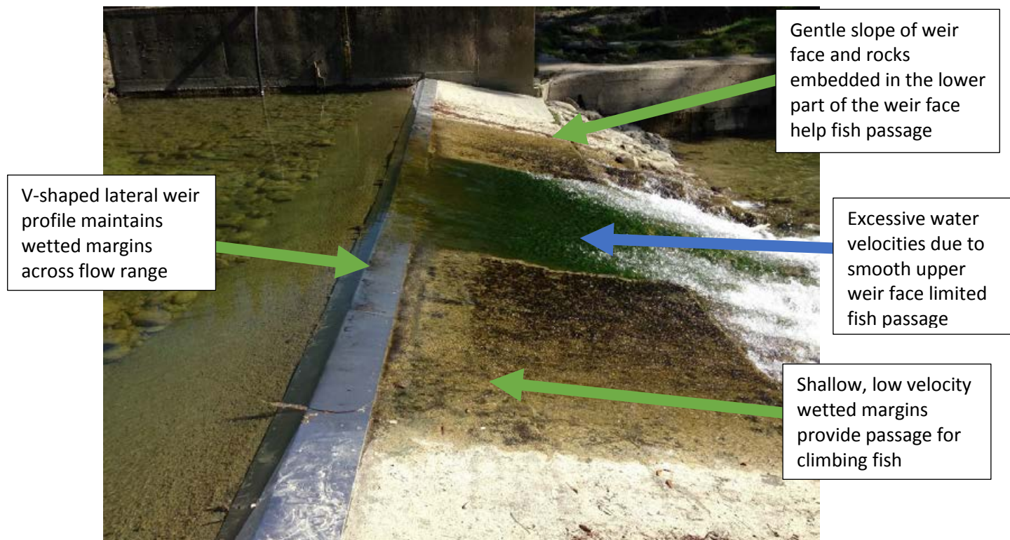
Figure E-19: An example of a crump weir used for hydrological gauging. Fish passage was impeded for swimming fish at this weir by the high water velocities. Climbing fish were able to use the wetted margins on each side of the weir to pass. Credit: Paul Franklin.
