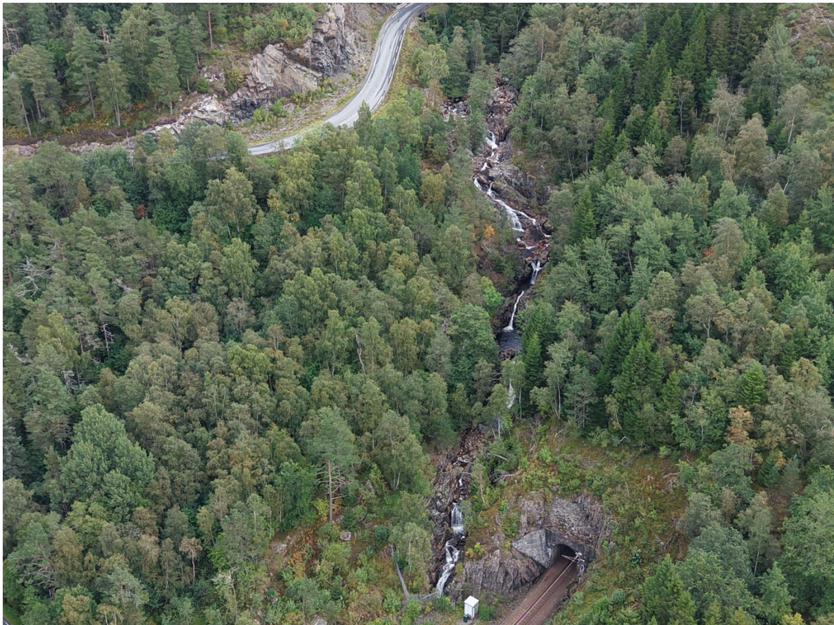
Figur 39: Fossen ca. kote 200-220 moh
