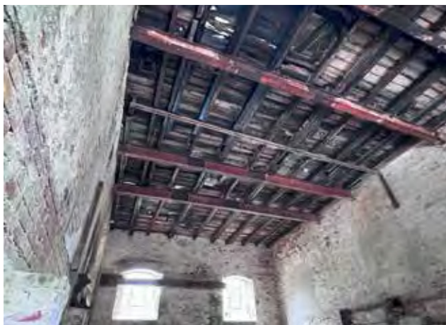
Sliperiet: Bjelkelag over turbinrom.
