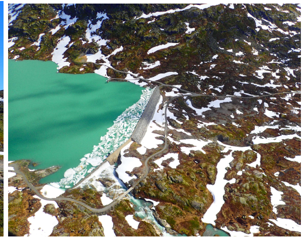
Dam Fivlemyrane i Luster Oppgradert i 2006 ny oppgradering > 2030
