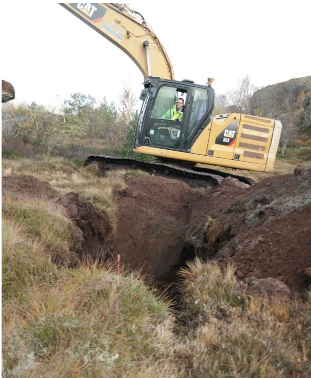
Figur 7 - Prøvegrop DEP4, gravedybde ca. 4,5-5,0 meter
