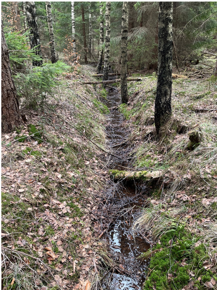
Figur 4-13 Dreneringsgrøft.
