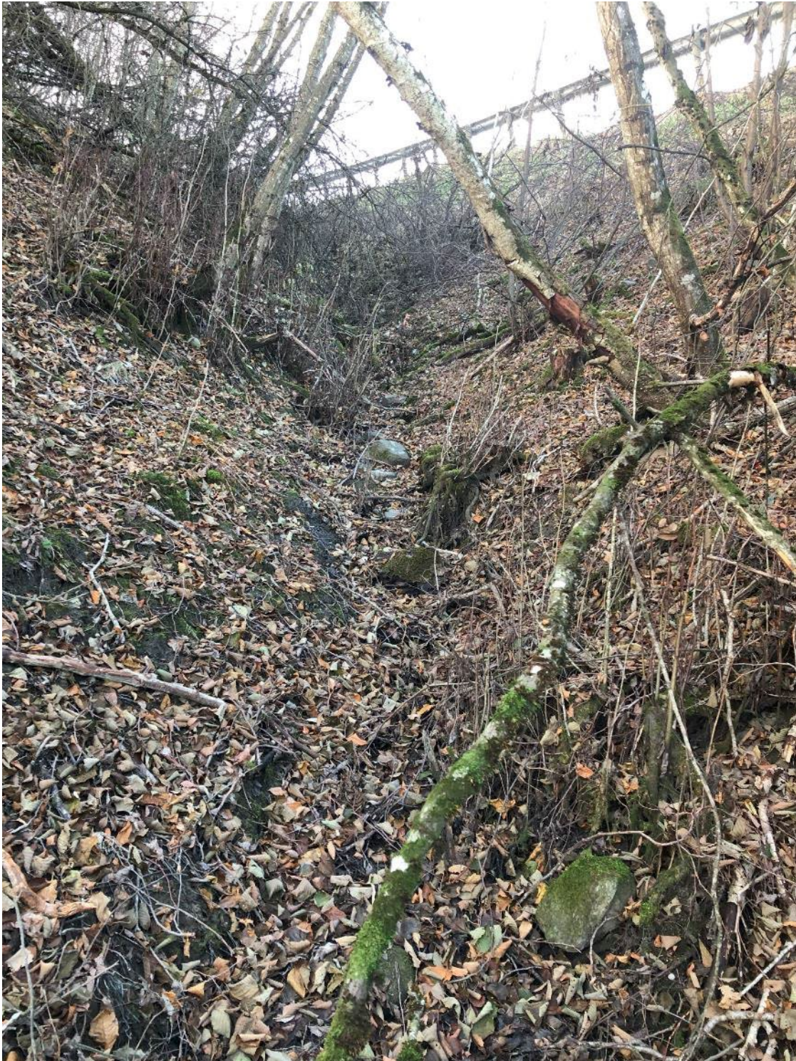
Figur 11 Ravine over tiltaket
