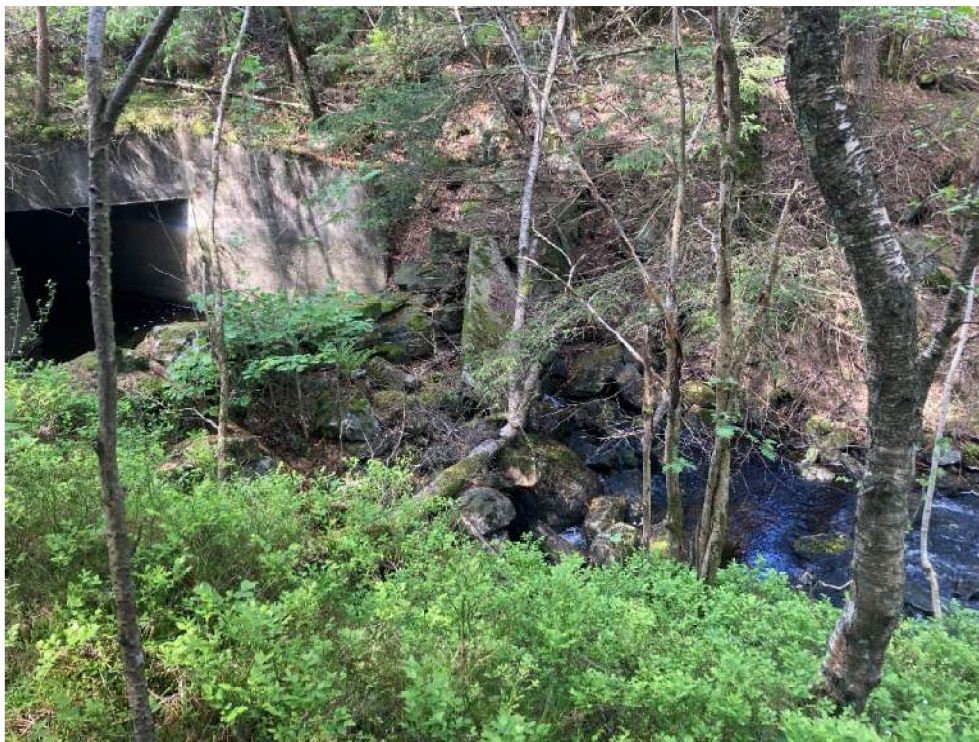
Figur 19 Eldre steindam like nedstrøms for fv 47
