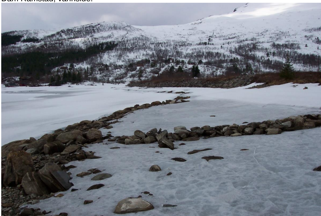
Dam Ramstad, vannside.
