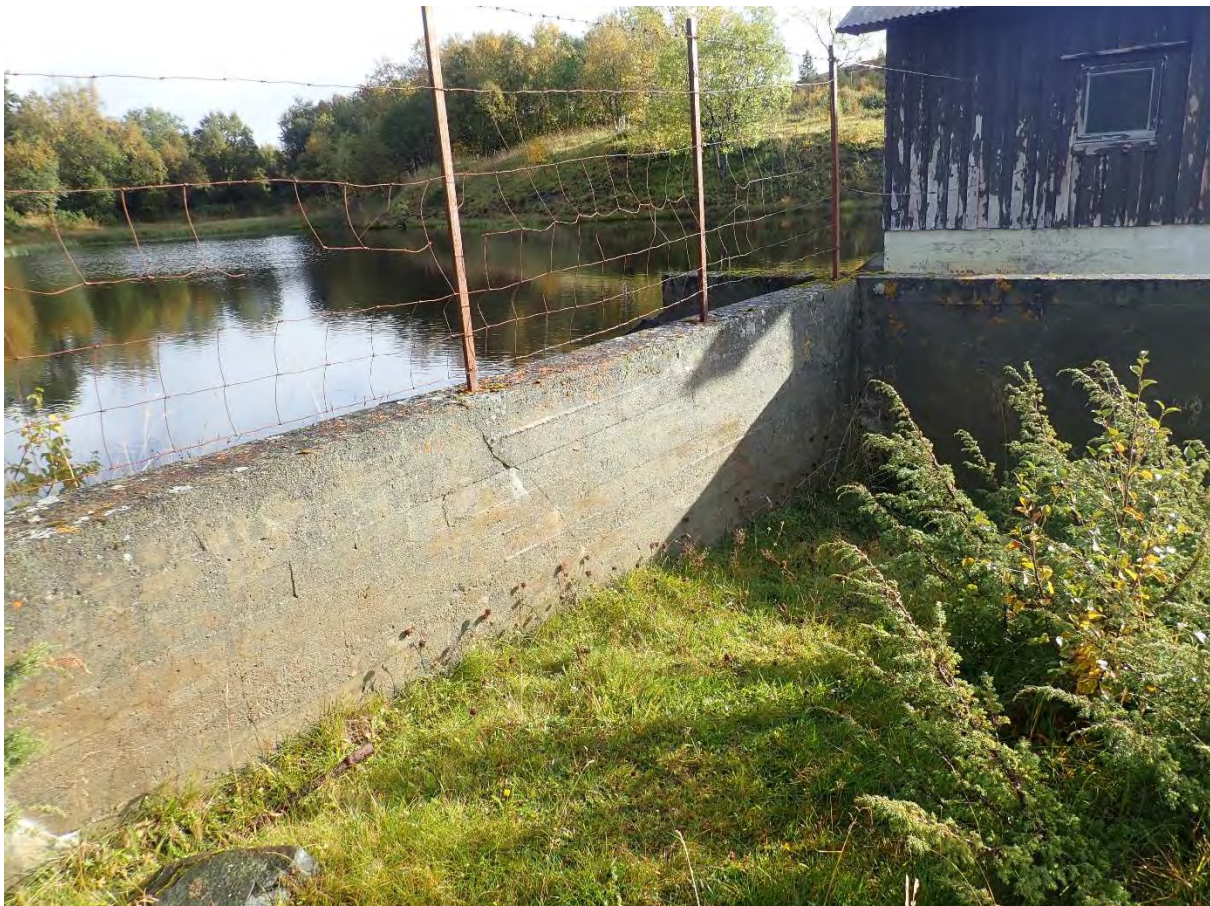
Figur 4. Betongtetting.
